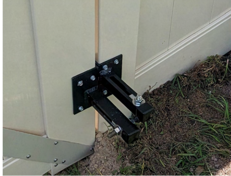
LOWER HINGE (PIVOT HINGE)
