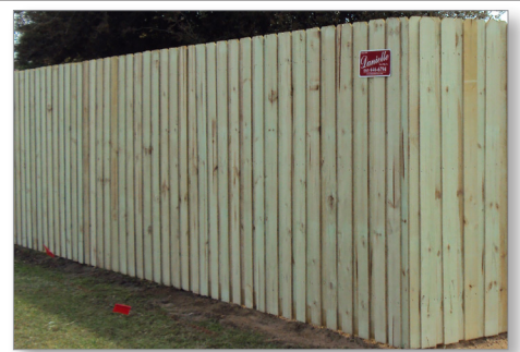
Water Sealed Board on Board - 6' Height
