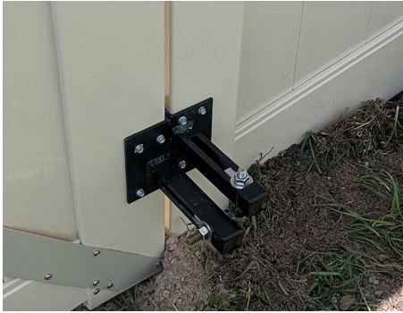
LOWER HINGE (PIVOT HINGE)
